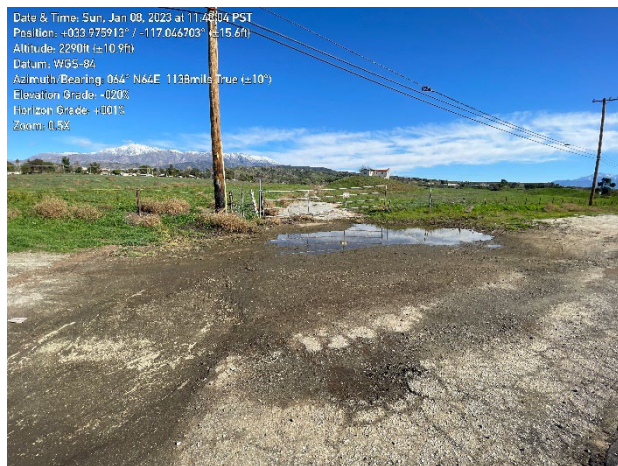
Ponding water in offsite area along Calimesa Boulevard, northwestern portion of site facing east-northeast (01.08.2023).
