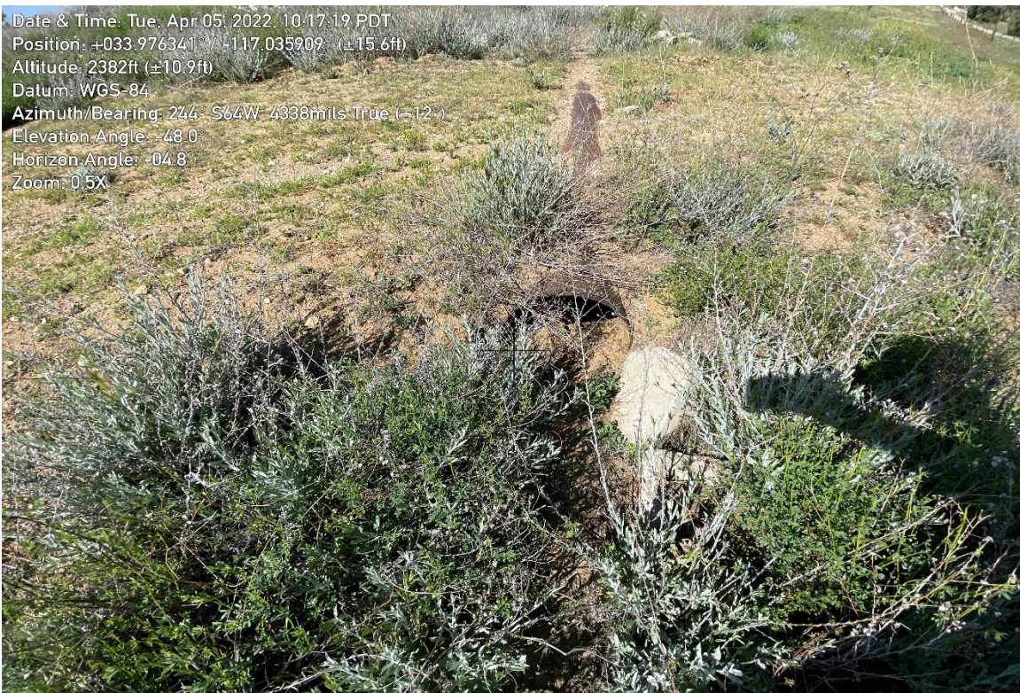
Portion of underground pipe, D4 facing southwest.
