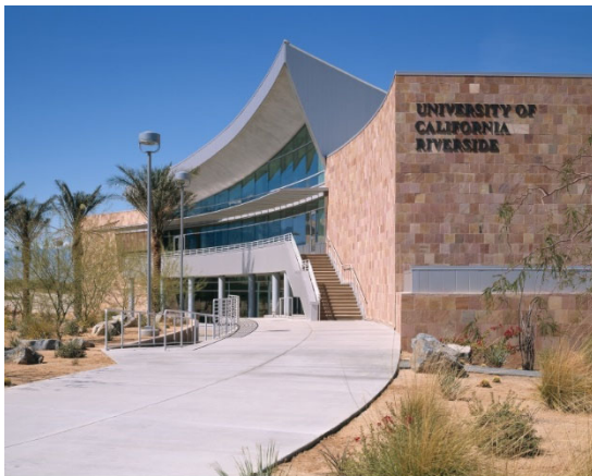
Campus Roof Variation
