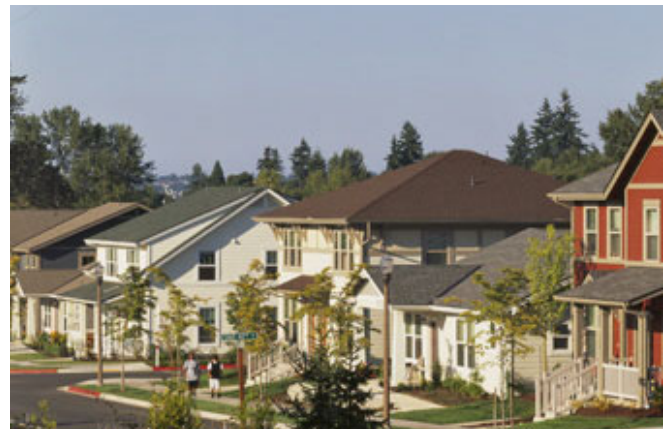
Different Elevations along Street
