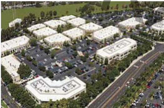
Office Landscaped Parking
