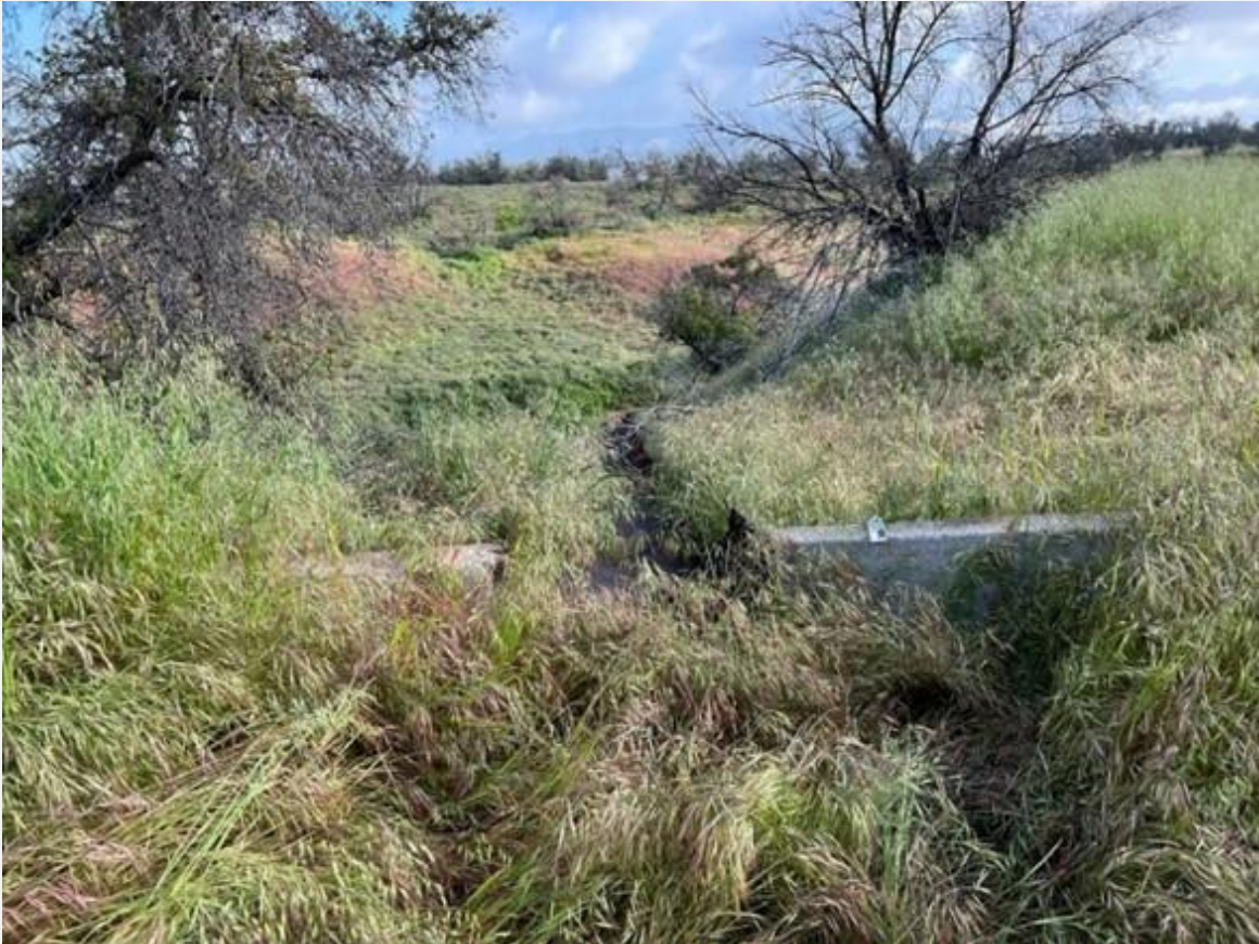
Figure 9. Overview MV-S-002, drainage pipe feature, facing north.
