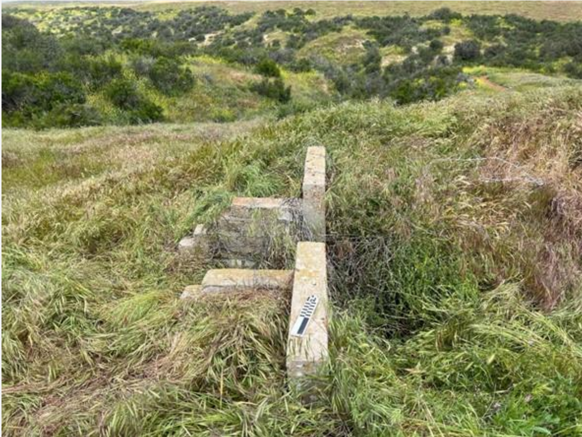
Figure 11. Overview of MV-S-004, drainage pipe feature, facing north.
