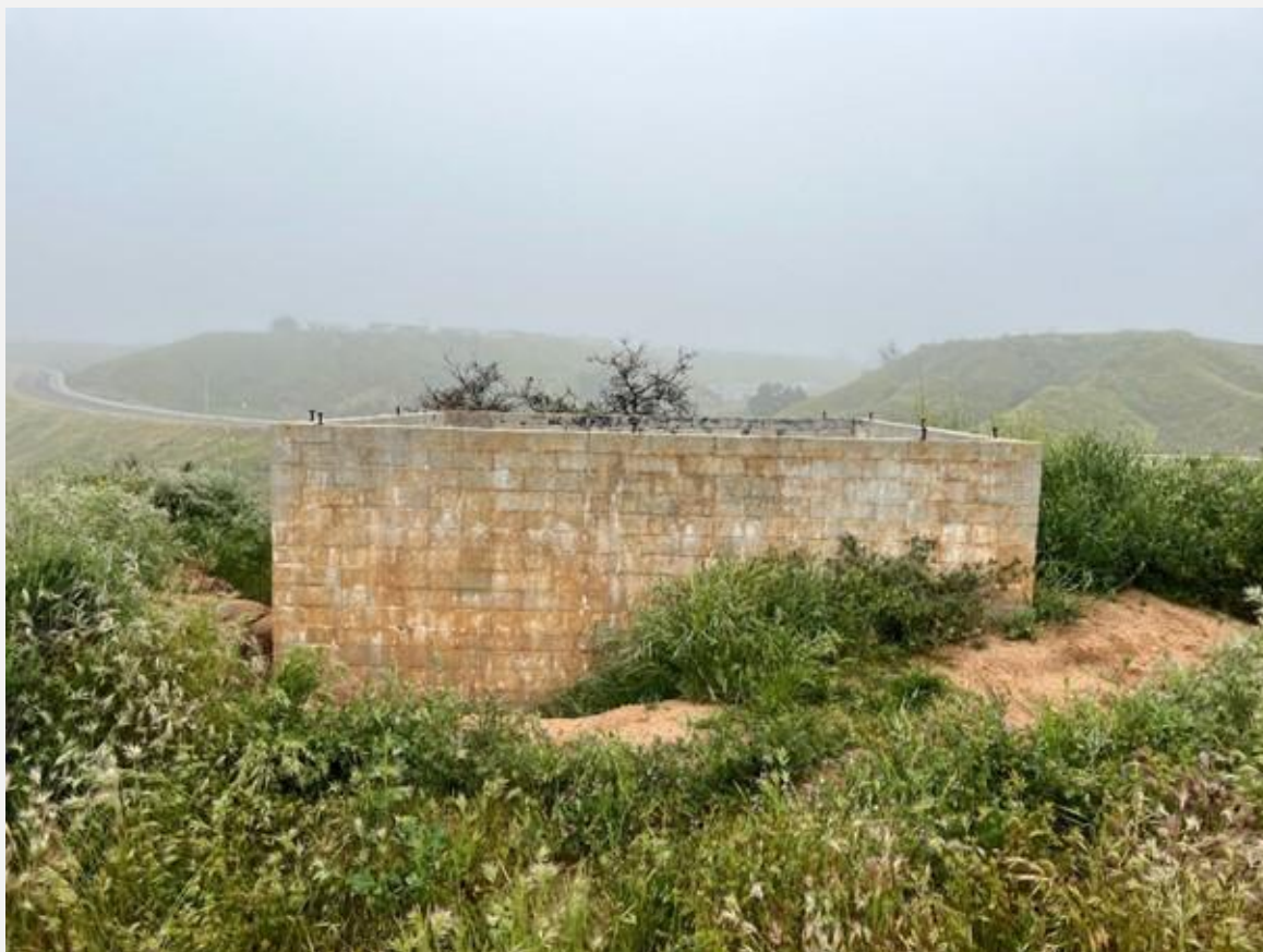
Figure 7. Overview of previously recorded P-33-013995, concrete reservoir, facing north.
