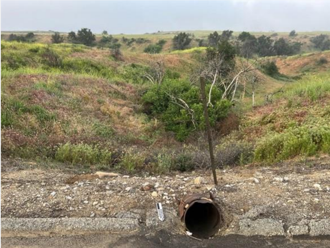
Figure 14. Overview of MV-S-007, drainage pipe adjacent to road, facing south.
