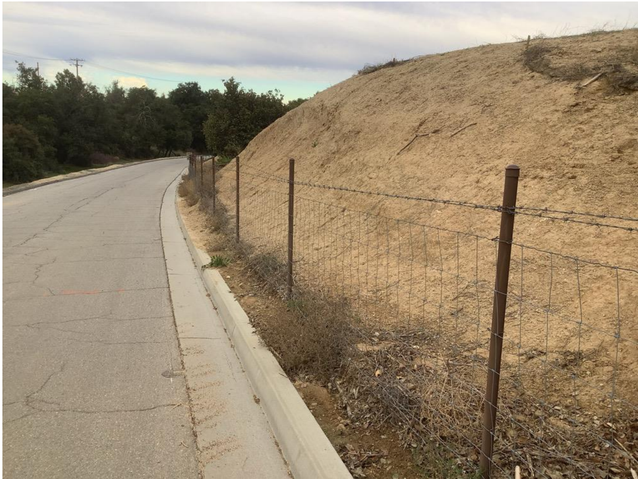
Photograph 8: Road cut exposure, approximately 15 feet high. Located on the north side of County Line Road just east of the water tanks. Sediments of the old axial channel deposits as mapped by Morton and Miller (2006a). (photograph taken by David Alexander, facing west).
