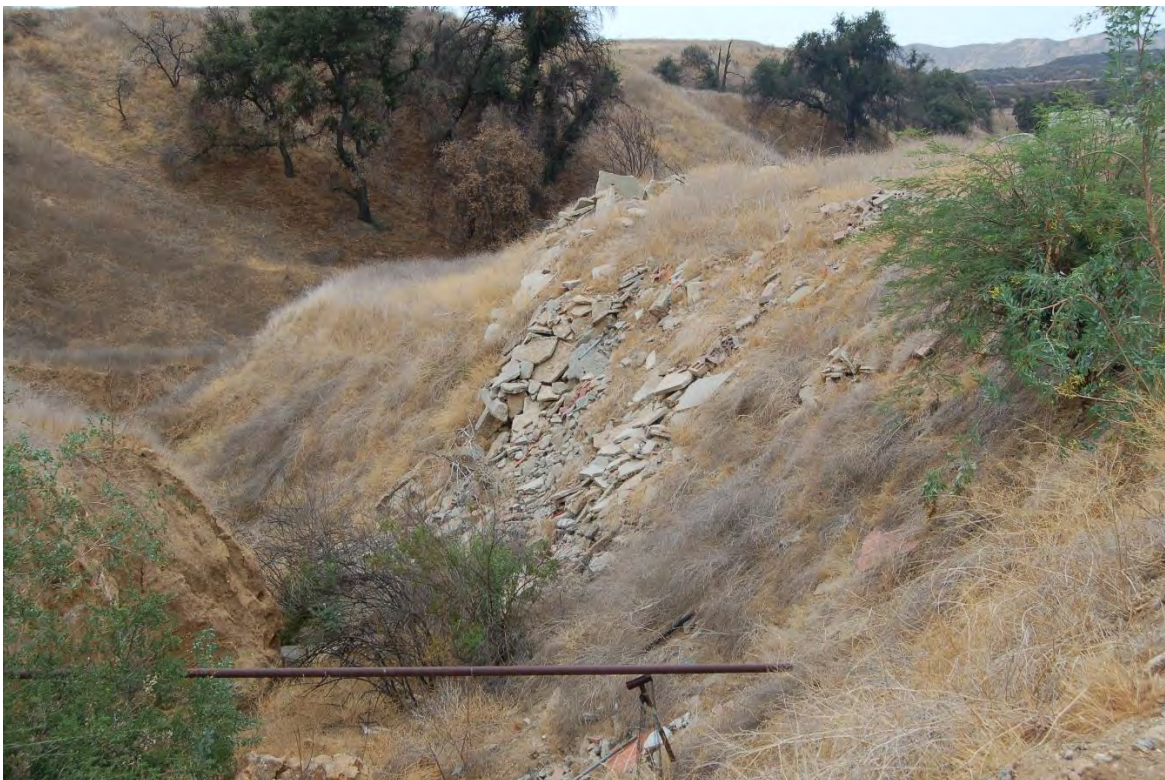
Photo # 4 – south view of dumped concrete, clay pipe, and brick in canyon south of the olive orchard in the northeastern portion of the Site. What appears to be a metal water line is visible in foreground.
