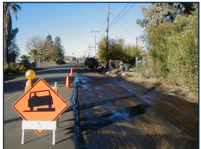
Road work on 7th Street is an example of the City's ongoing efforts to provide high-quality public infrastructure.
